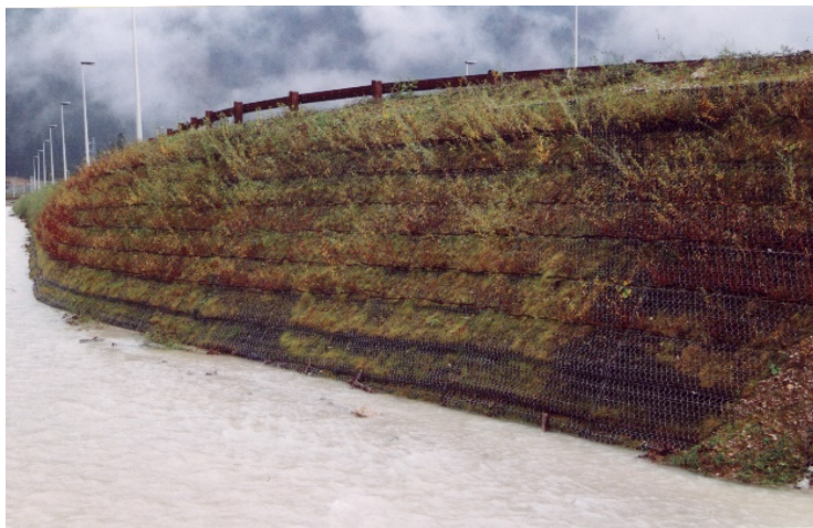
Fig. 1. Green reinforced earth Terramesh, 2000
