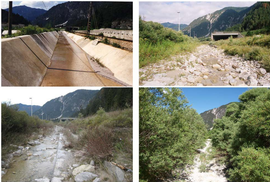
Fig. 4. Fella river ante operam (1998 - upper left corner) and post operam (2006 - upper right corner, 2009 - down left corner and 2017 - down right corner)
